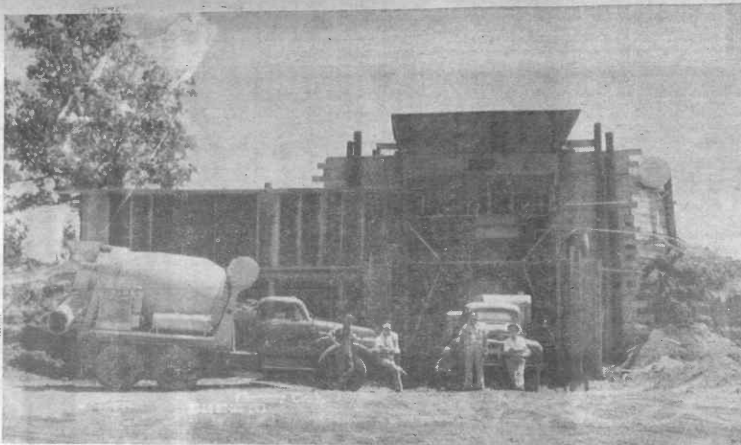
READY-MIX CONCRETE PLANT—Shown here is the recently opened Milligan Ready-Mix Concrete Plant on highway 25 north. Kell Milligan, owner and operator of the plant, states that he is
